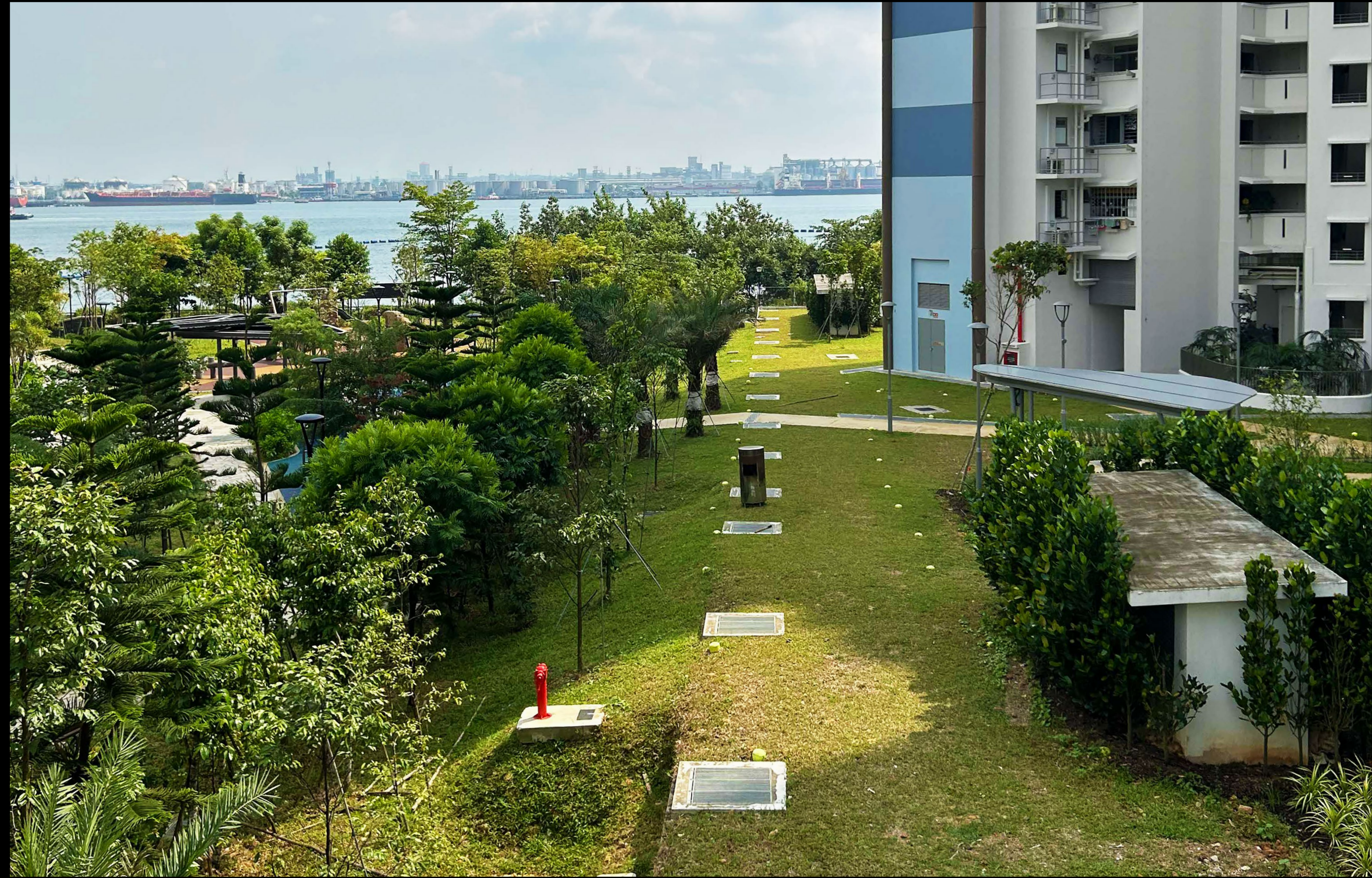
Detention drain system along the precinct's boundary
