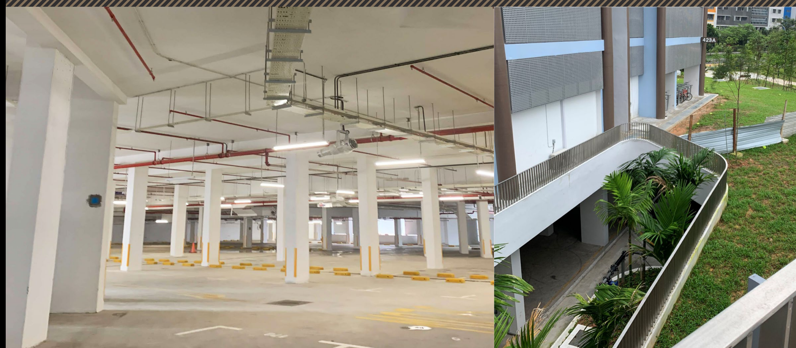
Maximising footprint of basement car park to reduce excavation works, simplifying earth retaining and stabilising structure system
